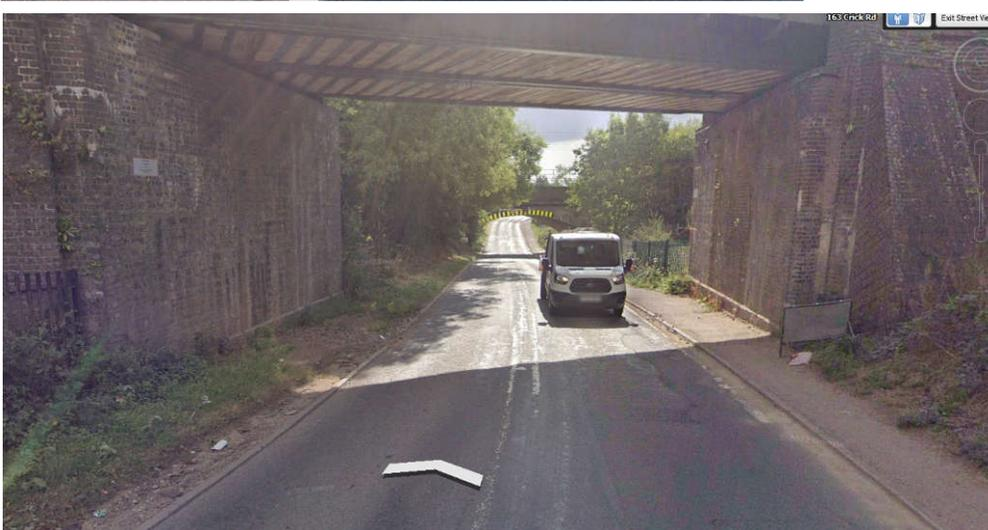
Appears to be sufficient width to re-locate motor-vehicle lanes approx 1 metre to the left and create a  $\approx 2\text{m}$  wide shared use path.
