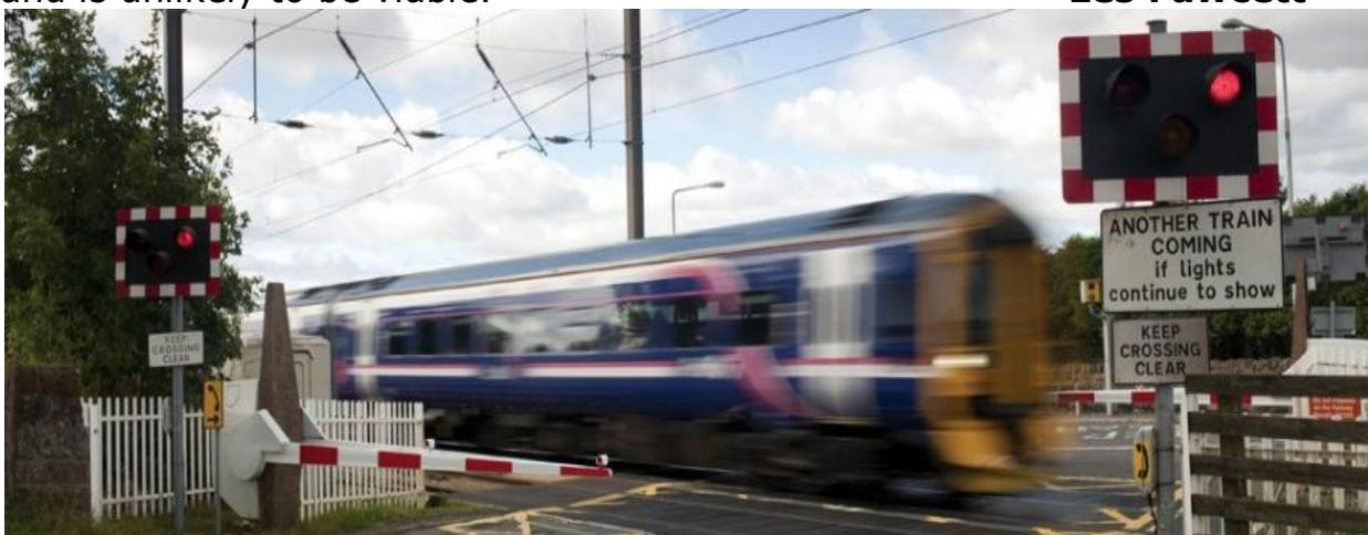
A typical British AHB level crossing taken from a recent article in The Rail Engineer.
