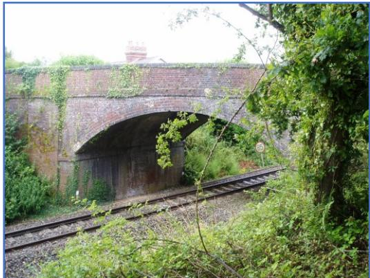
2) *Bridge 499 between Talaton & Whimble shows how the arch design may restrict clearances for double track restoration.*
