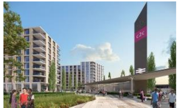
New c2c Beam Park station, between Rainham (Essex) and Dagenham Dock.
