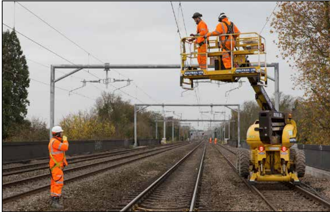
WORK GOES ON: Overhead equipment on the Barking-Gospel Oak line
