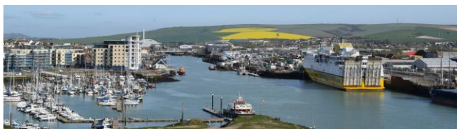
Newhaven-on-Ouse, East Sussex, looking north
