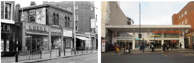
Dalston Kingsland station – site in 1966, new in 2017!
