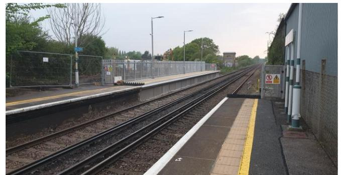
A near-complete extension of the up platform at Cooksbridge, to avoid 8-car trains fouling the A275 level crossing
