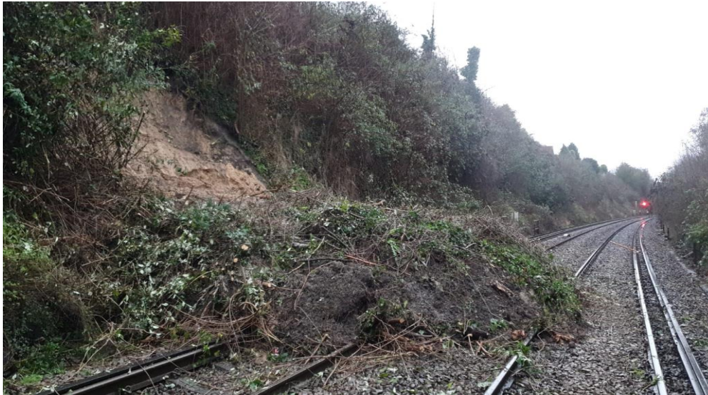
Cuxton Landslip – December 2019
