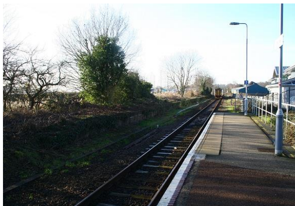
Fig.9. Former 'up' platform at Melton
