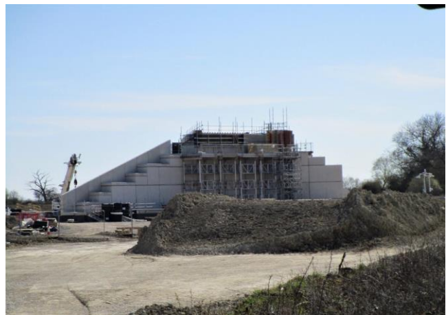
Launton The EWR route runs diagonally from left (west) to right while, in the centre, work continues on building a new overbridge for a realigned Station Road. The existing road is closed until mid 2022. New road overbridge under construction from ground level.
