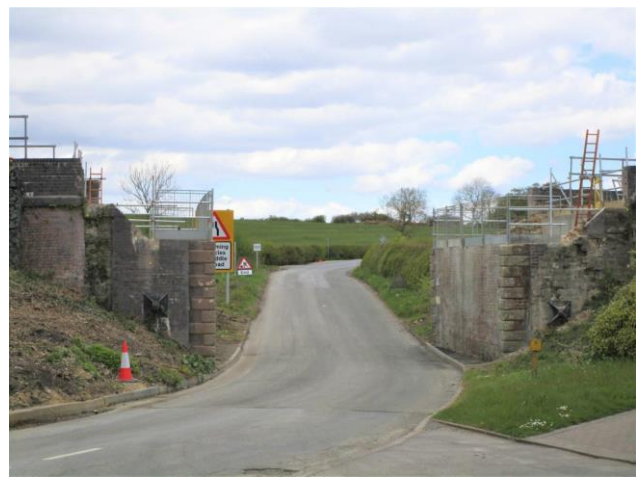
Marsh Gibbon/Poundon Large work site to the left of the former station site (middle right) with new temporary access roads for the east and west approaches. Yet another road underbridge that is being completely replaced. Marsh Gibbon/Poundon bridge abutments awaiting delivery of new bridge deck.
