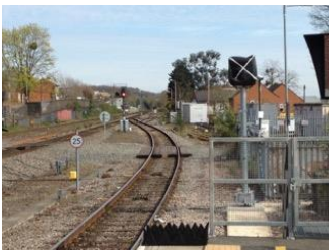
The new repeater signal at the end of platform 1 at High Wycombe has been installed. Unlike the signal at left it can be seen the length of the platform and will allow trains to use the full length thus reducing the long walk (twice as long for those connecting from the up platform). (Nigel Phillips)
