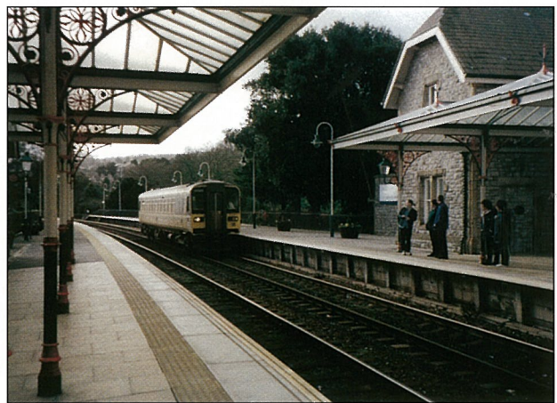
Grange-over-Sands: conserving the best of rails heritage
