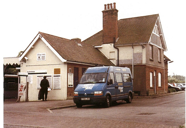
Southminster: from decay to rebirth. Construction work begins Photo courtesy of Essex CRP
