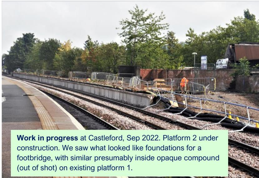
**Work in progress** at Castleford, Sep 2022. Platform 2 under construction. We saw what looked like foundations for a footbridge, with similar presumably inside opaque compound (out of shot) on existing platform 1.
