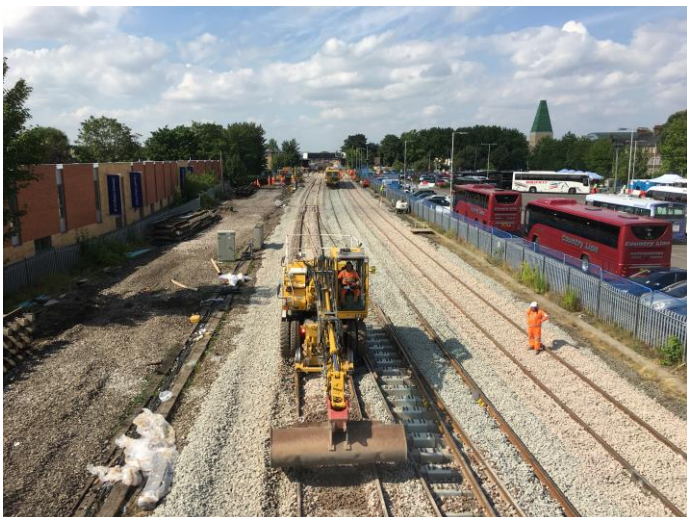
On Tuesday, looking north. Note new crossover.
