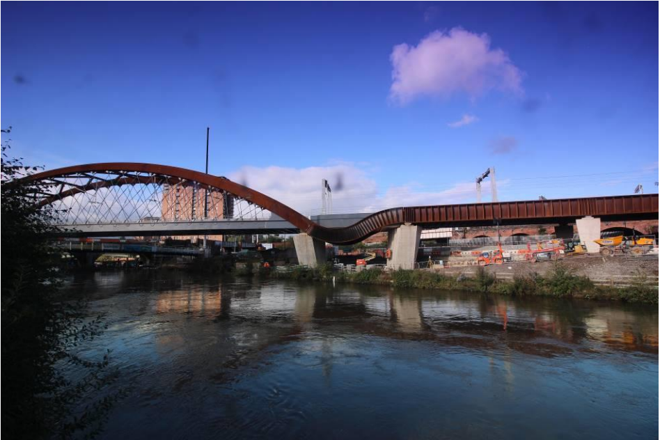
The new Ordsall Chord bridge over the river Irwell. This route is electrified, but it seems there may be few services making use of this electrification in the short term. Photo courtesy Network Rail.
