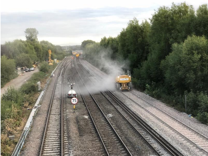
The new Down Oxford Relief line at Aristotle Lane.
