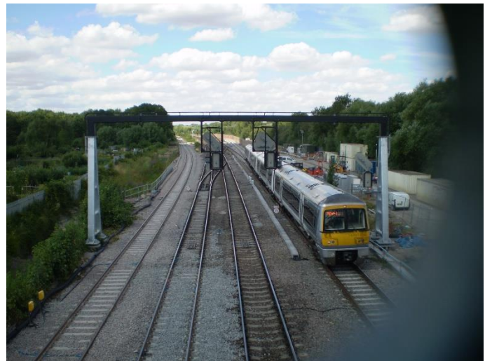
An Oxford bound Chiltern train comes off the new line, seen from Aristotle Road with the new Down Oxford Relief line on the left.
