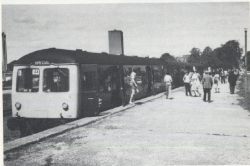
R.D.S. Special from Wisbech to Felixstowe on Sunday June 27th 1982 takes on passengers from the platform in Wisbech Goods Depot. (The passenger station was demolished shortly after closure). Photo: Peter Sumner
