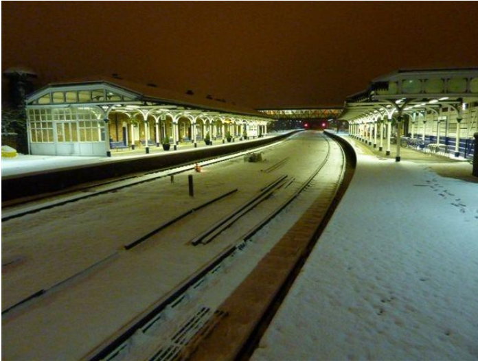
Selby Station on 28 November 2010: Services to and from London did not call here for over a week due to the extreme weather, although reduced services to Leeds, York and Hull were operated (photo - Selby & District Rail Users)
