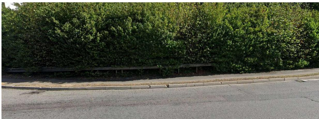
Also at this location, completely inadequate and poorly maintained pavement width, this is not even adequate for a single pedestrian, let alone for a bi-directional shared use path. Needs to be at least 3m wide.
