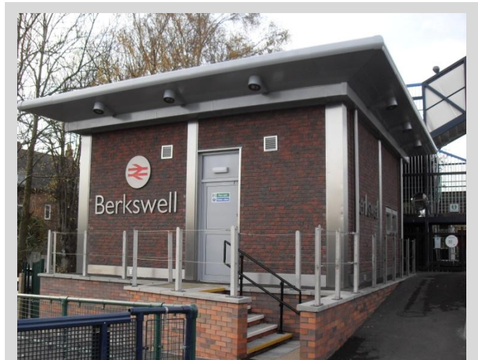
New modular station building
