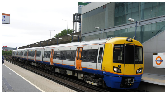
The modern London Overground station at Shepherds Bush
