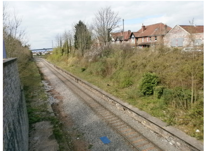
The existing Portbury freight line at Pill station will remain and a second track will be laid on the left for passenger trains to/from Portishead. Photo by Nigel Bray
