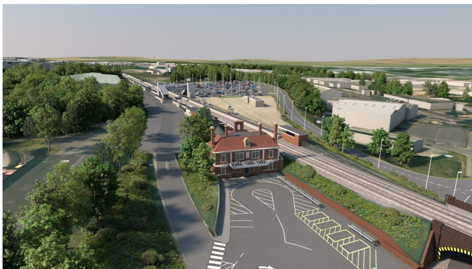
Realignment at Market Harborough will remove a severe speed restriction on the Midland Main Line. Image by Network Rail.
