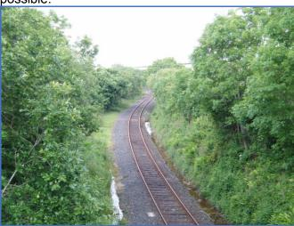
Photo 4. Looking north from farm overbridge 605. The platform would be on the left side. On the right the flooded section up to the middle of the picture is thought to be level track. Beyond, it is 1 in 88 down towards Crediton. (2012 photo)
