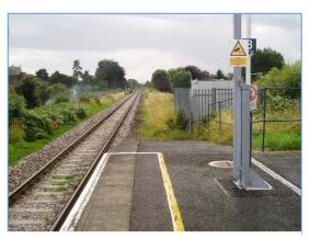
Photo 3. West from Whimple station. The existing former down line could become the through line and the old up line restored for trains stopping at the station.
