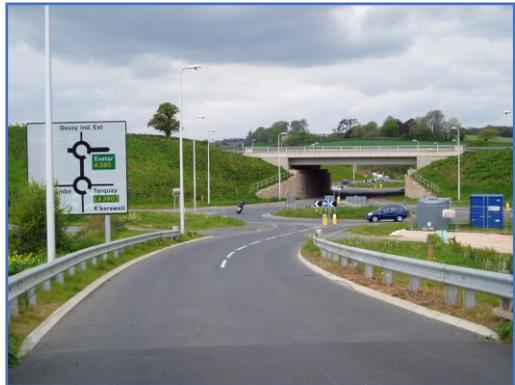
The chord on straight track could pass under the bypass road bridge in the background and on the left (south) side. It would be necessary to cut and divert the two roads leading left off the road sign. Continuing at 240 m radius the Plymouth line could be rejoined in about a ¼ mile (360 m) and to the south of the Old Kingskerswell Road bridge (railway location 215 m 46 c).
