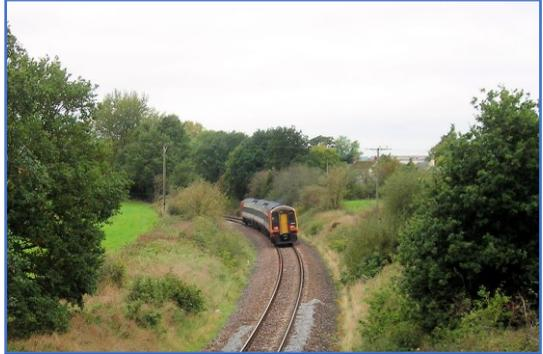
1) *The 12:20 Waterloo to Exeter St. Davids on 15<sup>th</sup> October 2018 recedes into the distance as it rounds the sharp curve at Talaton. All the way from Honiton to Pinhoe it was the down line that was retained, but here the track is swinging on to the up formation to ease the curve (on the right).*
