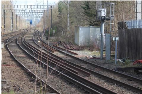
Fig.14 Looking north from Platform 3 at Cheadle Hulme. Wilmslow lines to the left. Stoke lines in the foreground. An new crossover is required between the up and down Stoke lines roughly in the position of the scrap rail in the picture.
