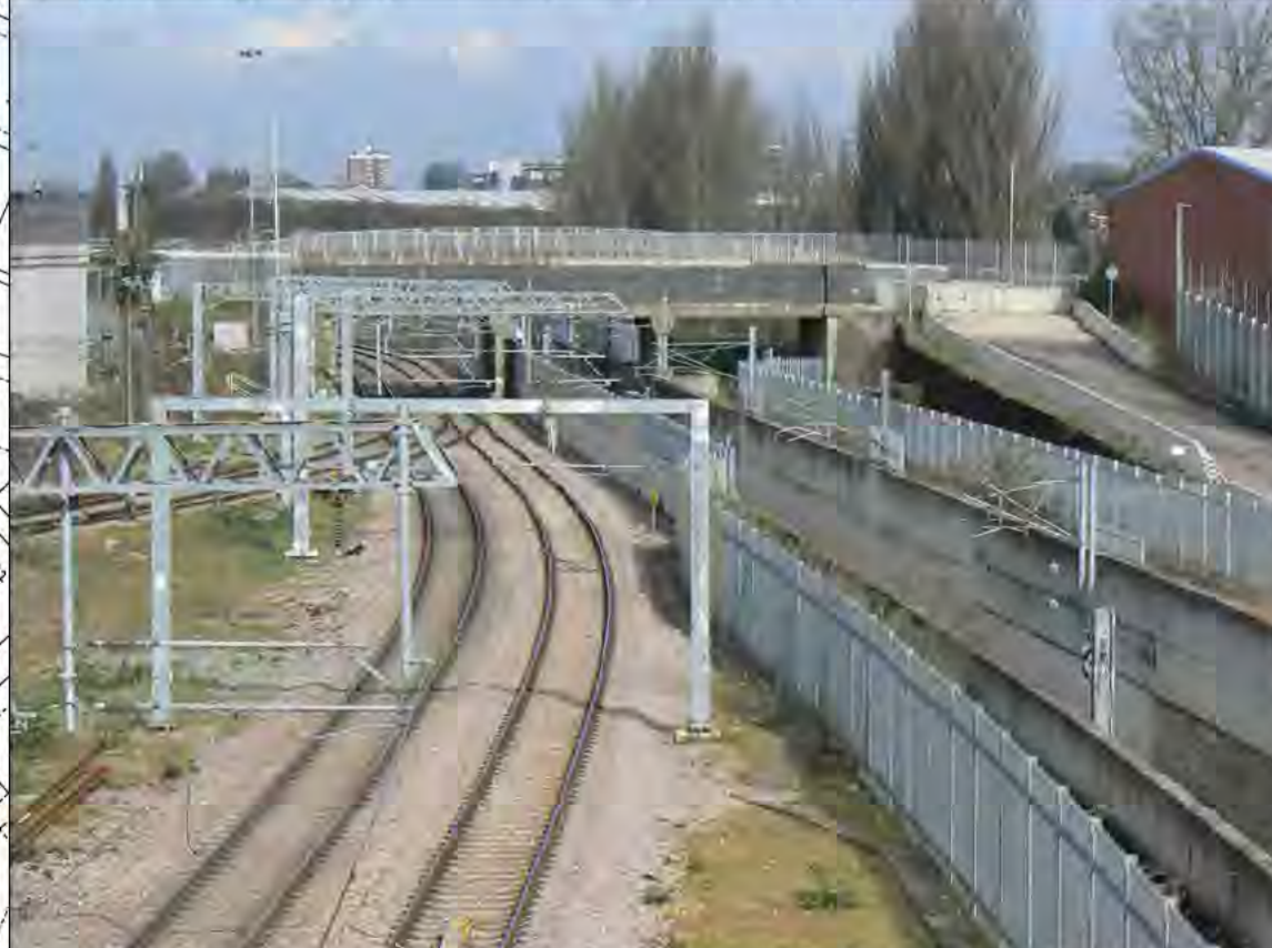
TEMPLE MILLS EAST JUNCTION AND STRUCTURE SDC 658
