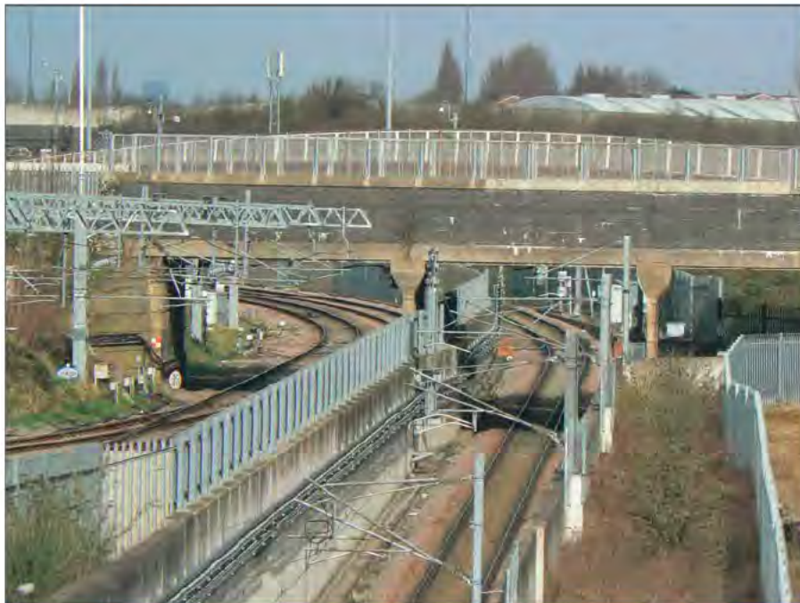
Figure 5.1 Overbridge SDC 658 looking north, Temple Mills East Junction on the left. Eurostar Temple Mills Depot connection on the right.
