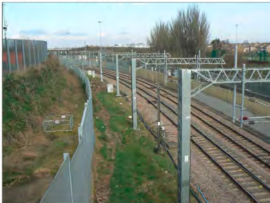
Figure 5.2 View from Temple Mills Lane overbridge looking north.
