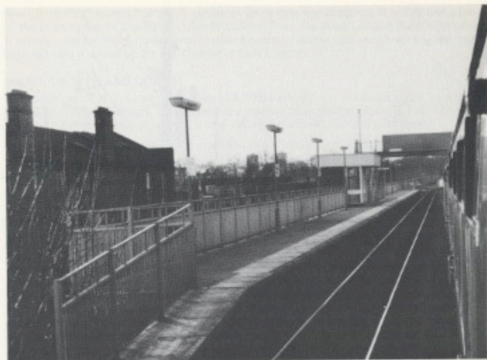
Hackney Wick Station reopened with G.L.C. funding on Woolwich - Camden Road Line Photo: W. L. Freitag
