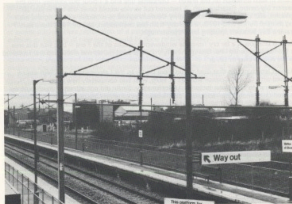
View looking north of the new station at Watton-at-Stone. (Reopened with local support May 1982.
