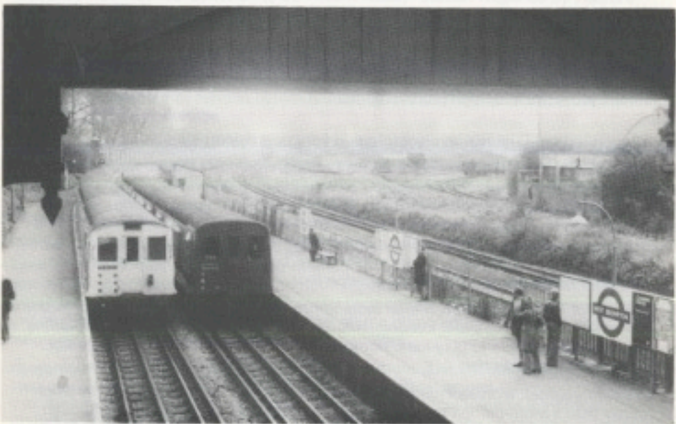
W. Brompton District Line with W. London Line running parallel
