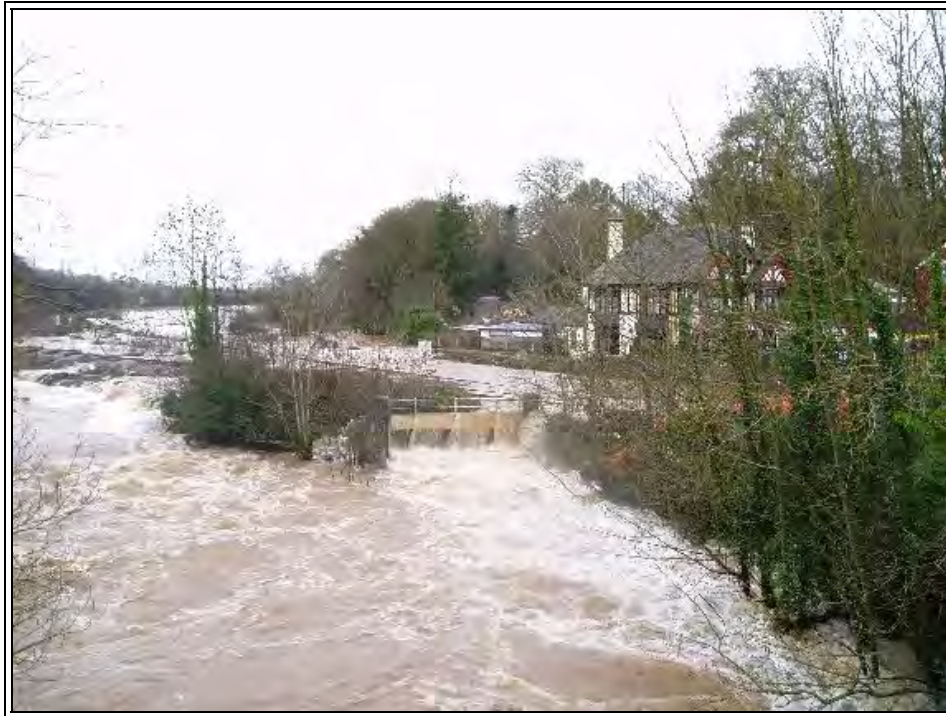
Figure 14. The main culvert at Cowley Bridge Junction overwhelmed by flood water on Sunday 23 rd December 2012.
