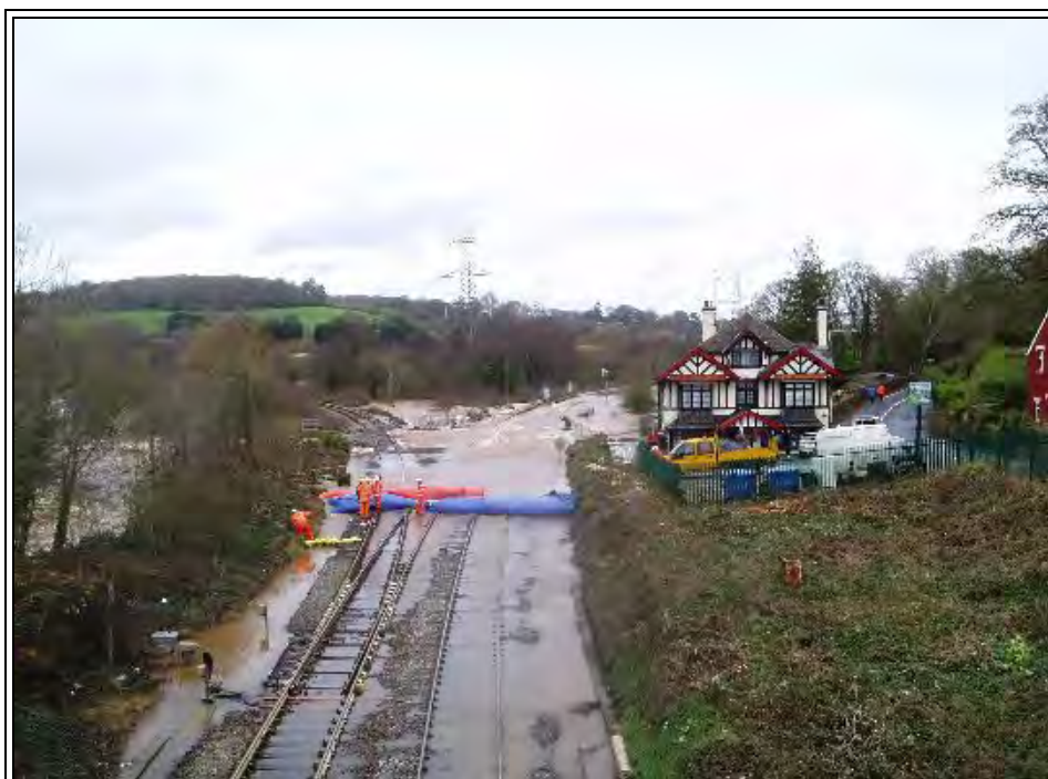
Figure 15. Cowley Bridge Junction overwhelmed by flood water on Sunday 23 rd December 2012.
