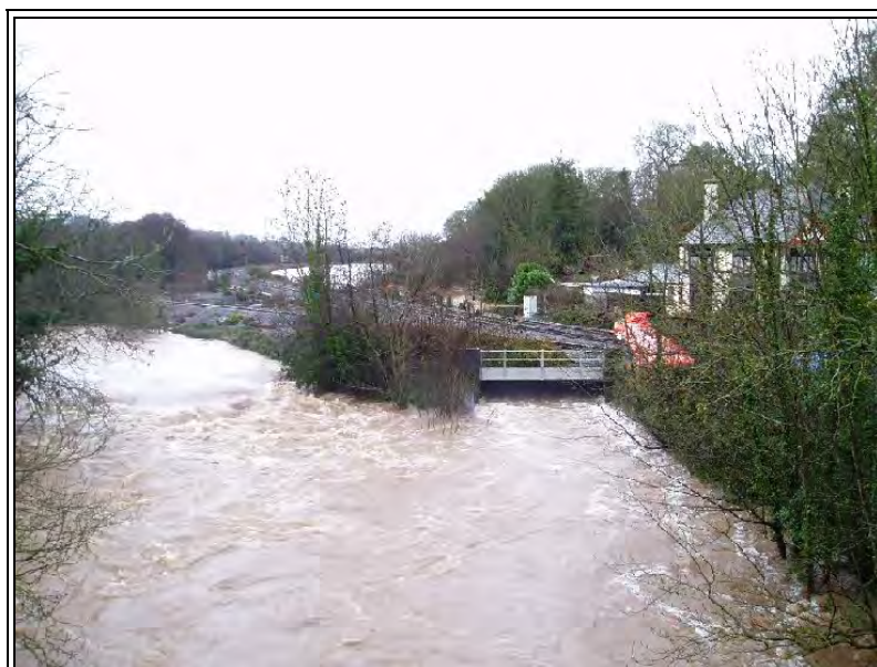
Figure 13. The main culvert at Cowley Bridge Junction on Saturday 22 nd December 2012.
