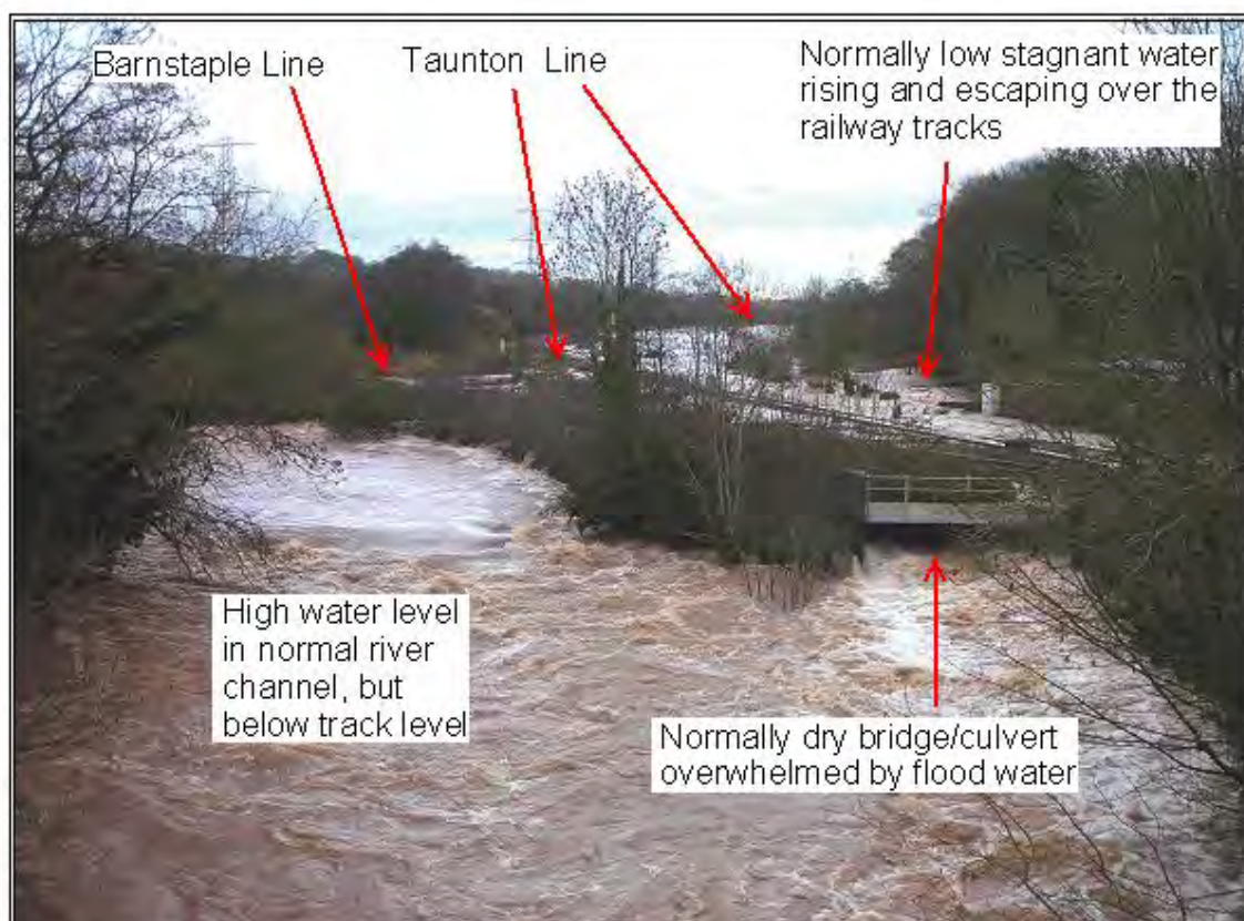
Figure 2. The River Exe at Cowley Bridge on 25 th November 2012 after water levels had begun to drop at around midday. The view is to the north close to the railway junction and shows the trapped water on the east side of the railway.
