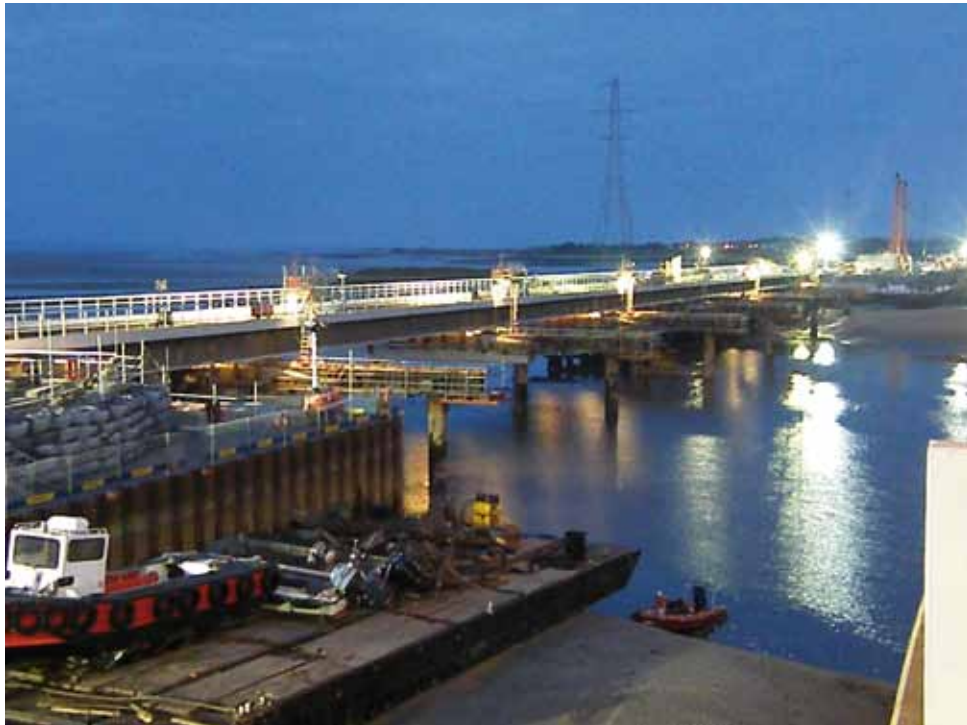
Picture: NETWORK RAIL
