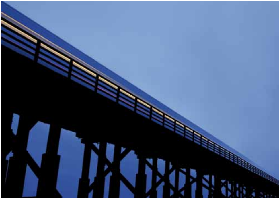
Picture: NETWORK RAIL
