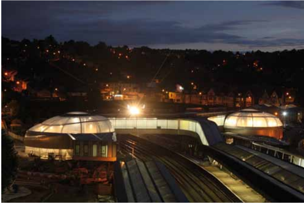
Picture: NETWORK RAIL
