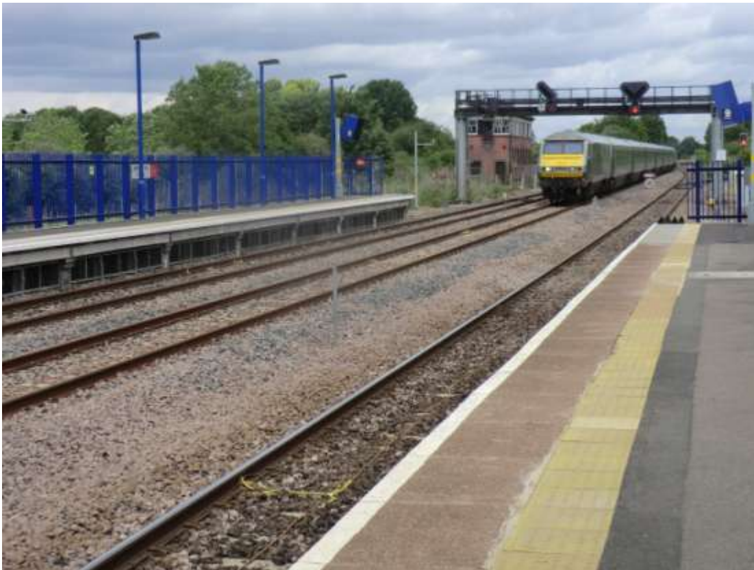
Chiltern platform extensions (for 9-cars) seen at Princes Risborough as the 11:12 from Birmingham speeds through on 17/07/15.
