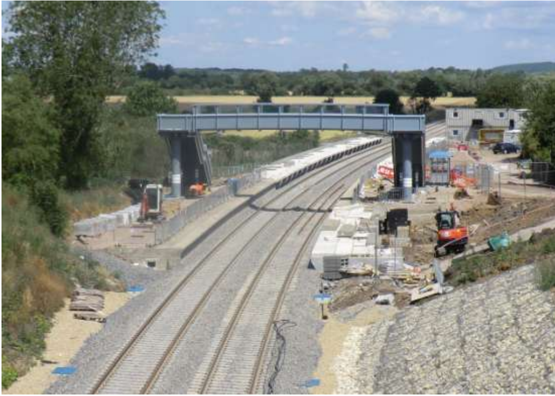
Islip station (looking east) nearly complete
