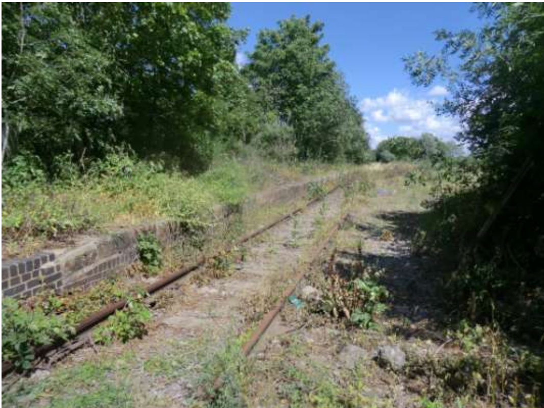
Looking east at the site of a proposed new Claydon station showing platform of the original closed in 1967. Note trackbed clearance to facilitate ground survey work
