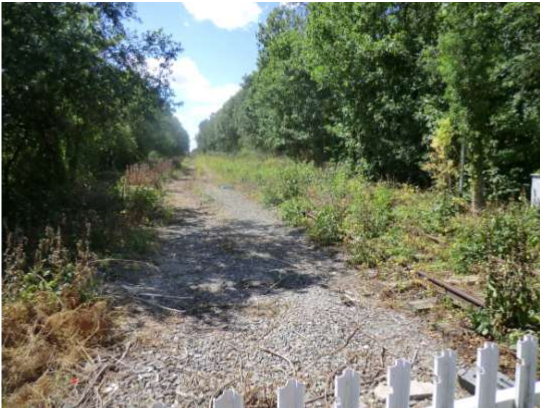
At Steeple Claydon crossing looking west showing trackbed clearance
